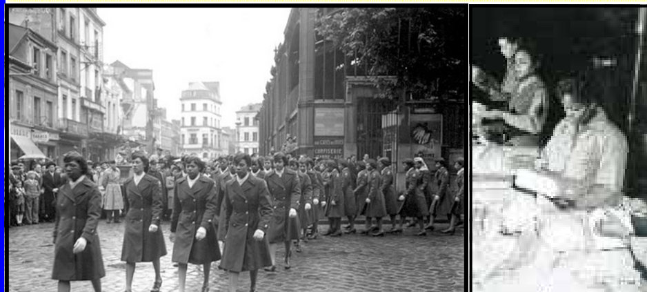
(L) Members of the 6888th Central Postal Directory Battalion take part in a parade ceremony in honor of Joan d' Arc at the marketplace where she was burned at the stake. 1945 The all-black 6888th Central Postal Directory Battalion arrived in England and performed its duties with distinction. Accustomed to discrimination at home, the women were accepted socially by British and French people.
